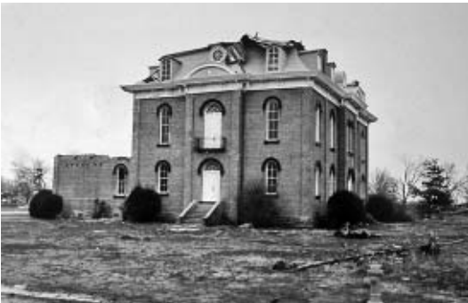
Damage to Jacksonport Courthouse from March 1, 1997, tornado (Photos by Mark Ballard)
